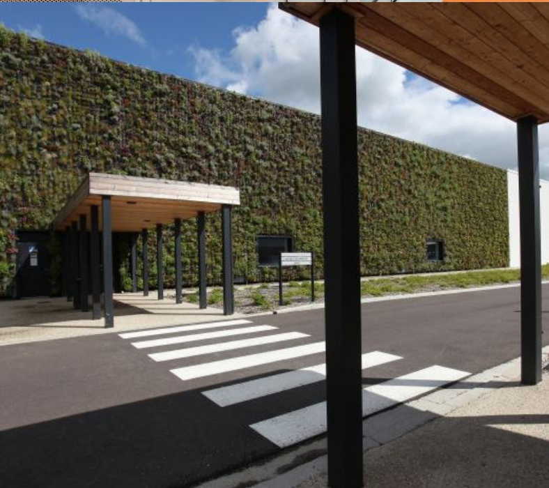
DATA CENTER ©ORANGE
