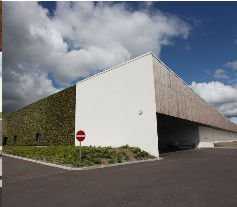
DATA CENTER ©ORANGE
